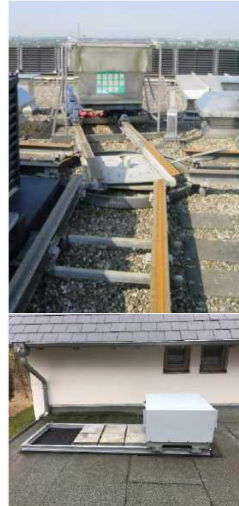
Frame Construction: partly stationary (Examples)
